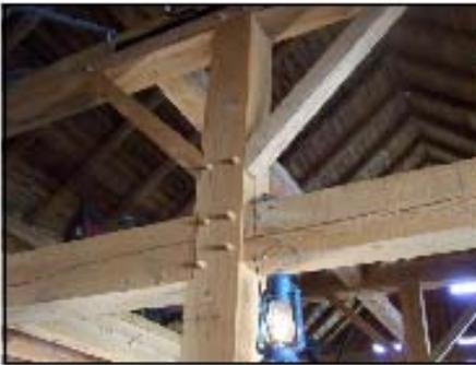
Often, in the case of a larger piece of furniture (or certainly a barn), or with any joint at an angle or where clamps can not be easily applied draw boring is the way to go. Glue is optional and in many cases would not have been used or relied upon.
