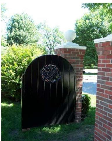
**Erl Poulin:** Fence Gate made from popular, fir and wrought iron and weighs 250lbs
